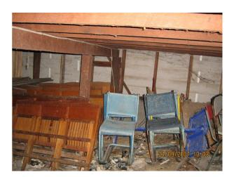
Under stage area – Remove items. This should not be used as a storage area for fire prevention and manual handling issues. Access doors to the area should locked, and the area assessed against confined space requirements and managed appropriately.
