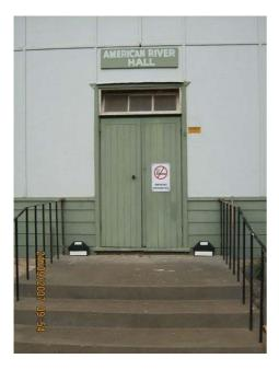
Front entrance – Ensure doors a structurally sound and weather proof. Replace door handle to comply with Emergency Exit door handles.
