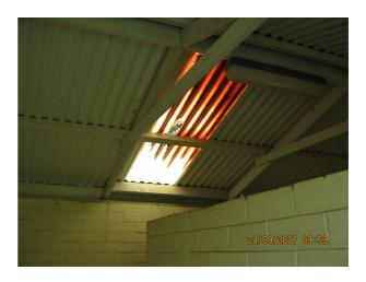
Skylight in toilets – Replace broken sheeting And install wire mesh under the sheeting to prevent a person falling through.
