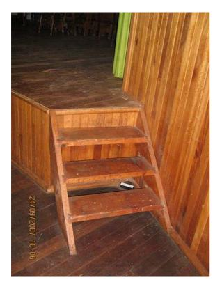
Stage Stairs – Install a handrails fixed to the wall, and non slip tread nosing to stair treads to both sets of stairs.
