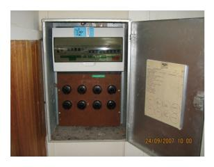
Electrical – Ensure Residual Current Devices protect all power points, and electrical equipment / appliances are tested annually by an electrician.
