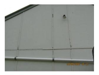
Exterior – Repair or replace broken battens.
