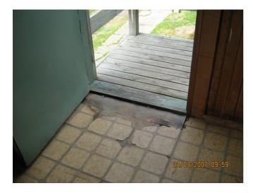
Flooring - Repair or replace vinyl floor covering, and install weather strip to door to prevent storm water from running under the door.
