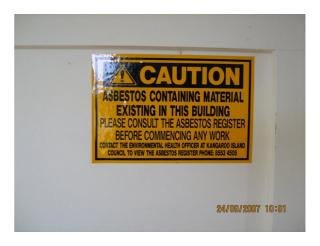
Asbestos Register – Ensure the Asbestos Register is located on site, and the register and asbestos products reviewed annually for changes / deterioration.
