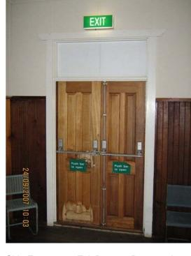
Side Emergency Exit Doors - Remove the rope from door push bars, inspect and service/repair Emergency Exit Doors and push bar mechanism to ensure the doors are able to be easily opened with minimal force.
