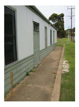
Side doors - Ensure doors are structurally sound and weather proof. As an interim measure assess the suitability and legality of providing a disability access ramp to a side door.
