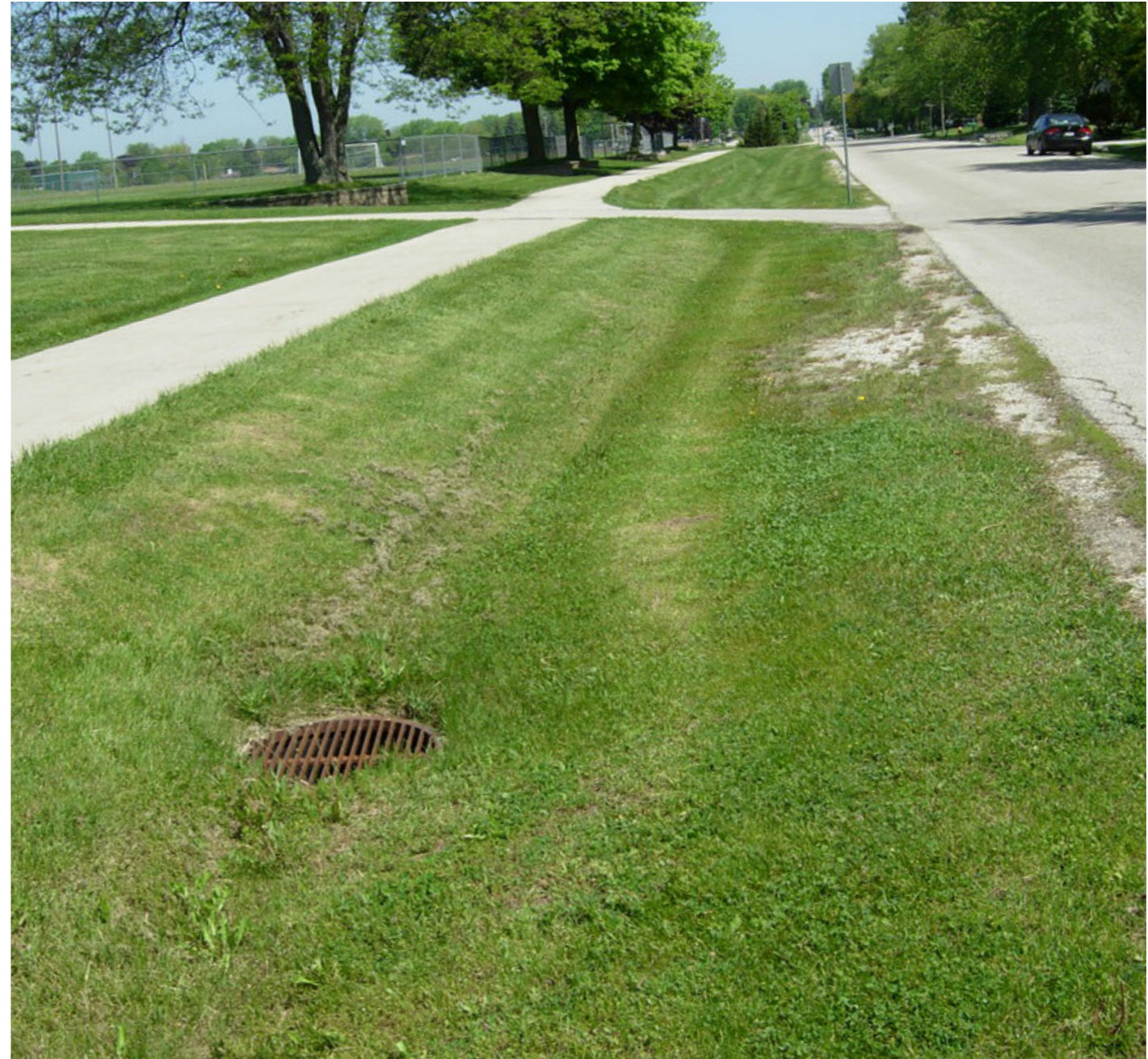
Passive drainage - swales with drainage, flush footpath and road
