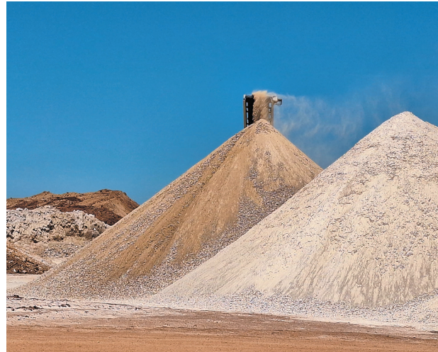
Stockpile of crushed material ready for spreading on Millers Road
