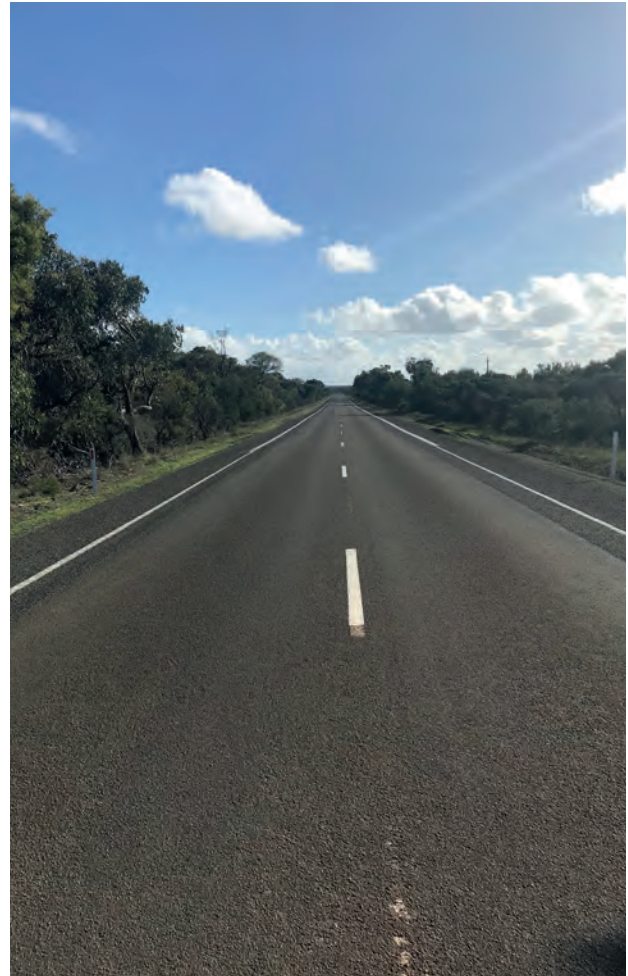
Shoulder seal completed on the Playford Highway.
