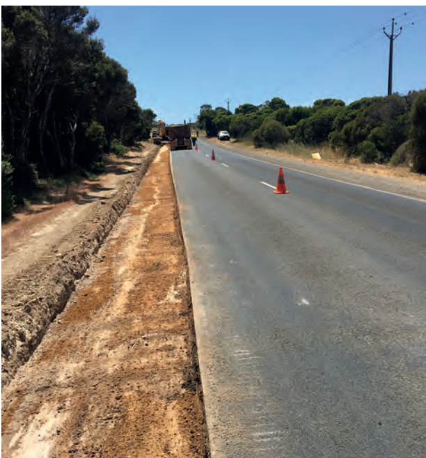
Preparation works before sealing the shoulder of Playford Highway.
