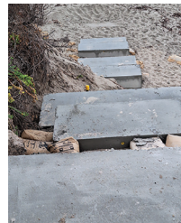
Footings (lower section) awaiting stair assembly
