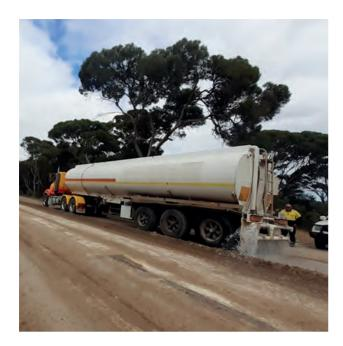
One of the two water trucks trialled by Council to improve grading of unsealed roads.
