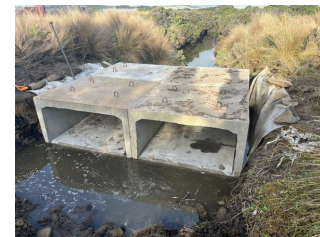
Pedestrian culvert crossing works in progress
