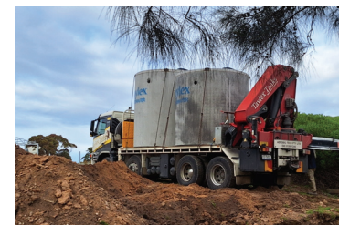
Delivery of Wastewater Treatment System
